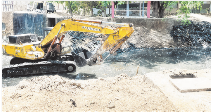
Heavy excavators deployed by BMC carrying out large-scale drain desilting.
